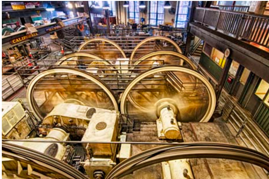
Cable Car Power
