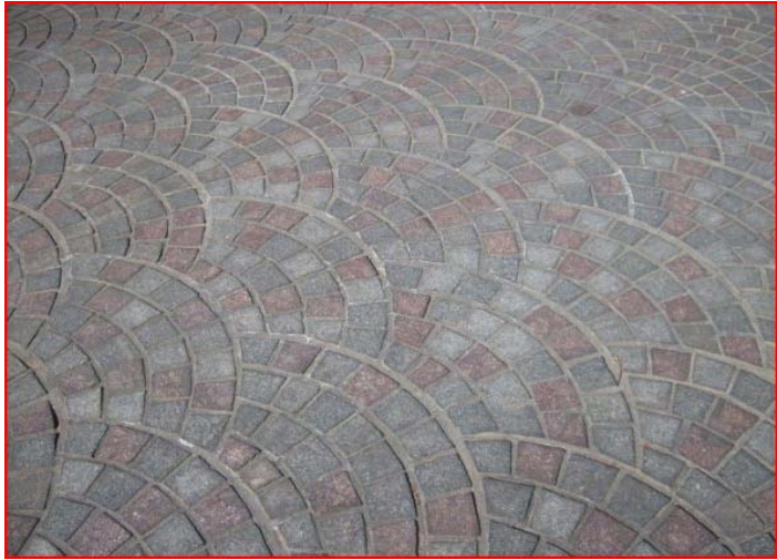
Porphyry, note how perfect installation is Possible with the preset elements
