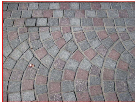
Porphyry, note how perfect installation is Possible with the preset elements
